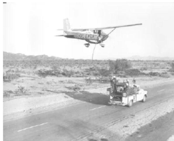
The Hacienda Cessna 172 refuelling during its record flight. Source: McCarran Airport
