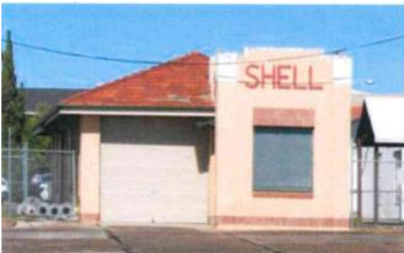
Figure 1: Northern elevation of the Shell Kiosk (AHS 2021).
