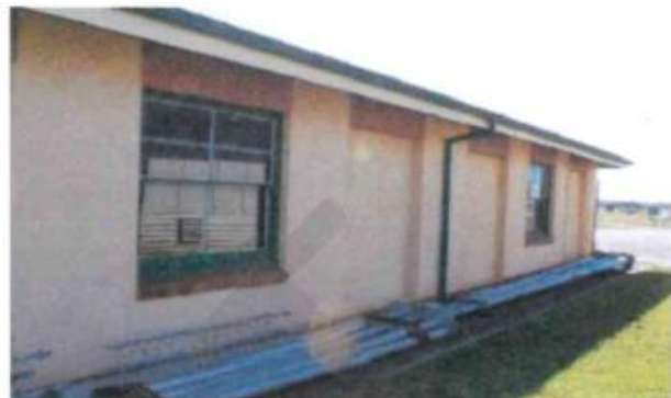
Figure 2: Eastern elevation of the Shell Kiosk (AHS 2021).
